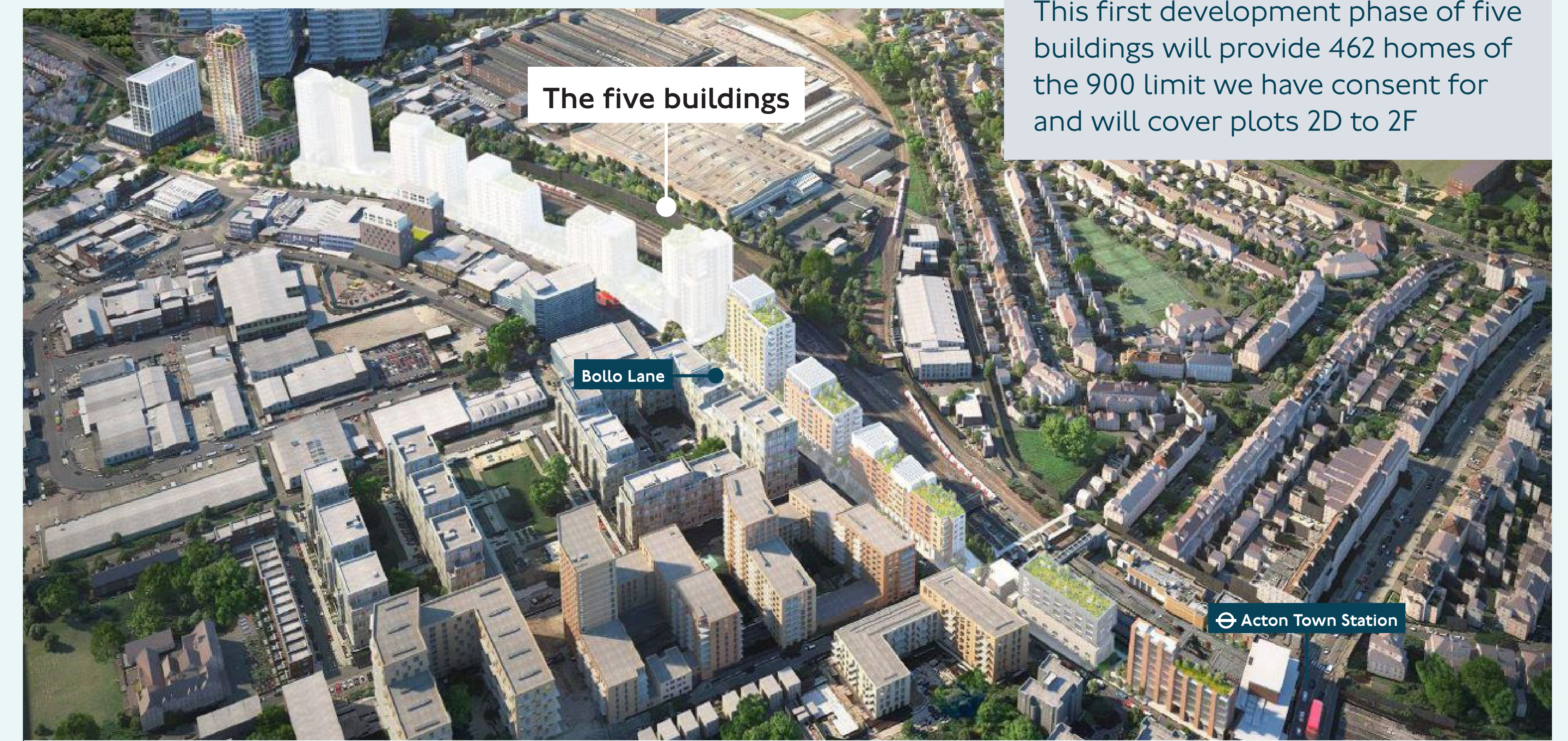
Aerial view showing the five buildings (plots 2D to 2F) with new design detail
